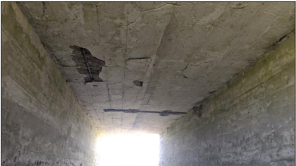
Figure 3. McLarty Line over Fields Creek Drain – Interior Culvert Surfaces, showing severe delamination and spalling with exposed corroded rebar, as well as an observed Barn Swallow nest
