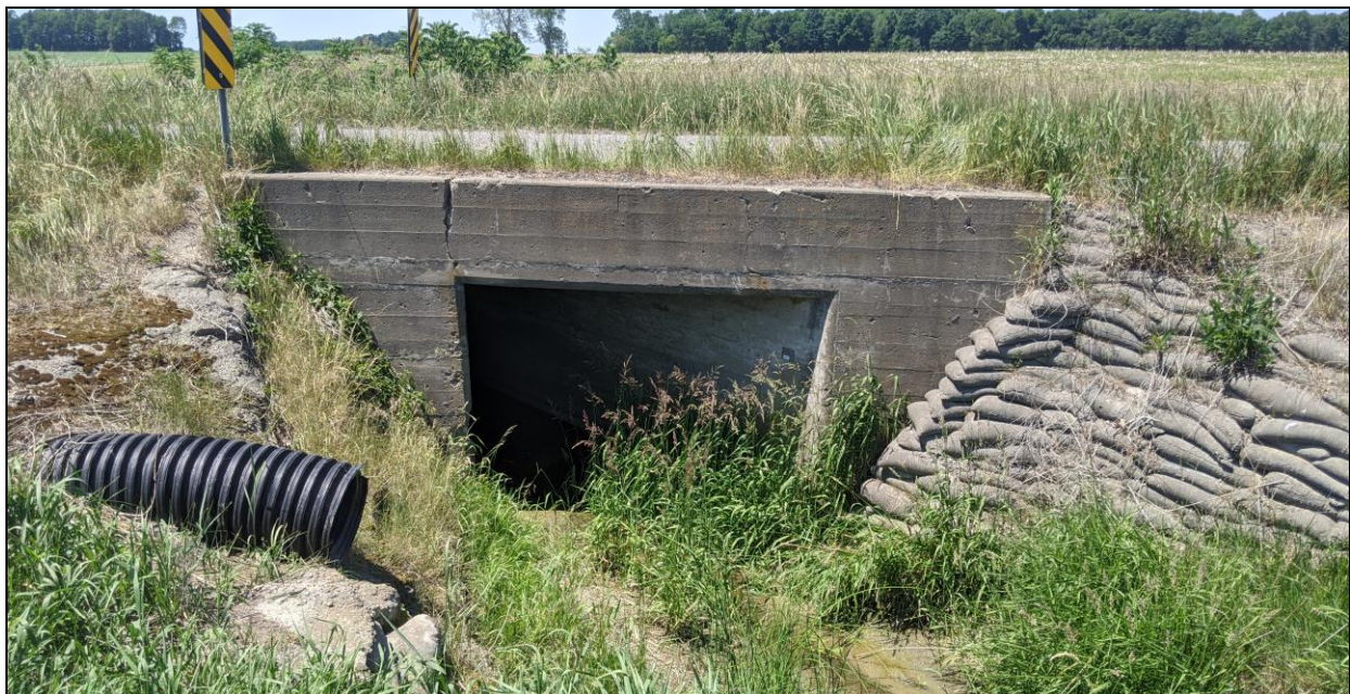
Figure 1. McLarty Line over Fields Creek Drain – South Culvert End, showing structural movement cracking on culvert end wall and fascia, and deteriorated state on “concrete bag” retaining walls
