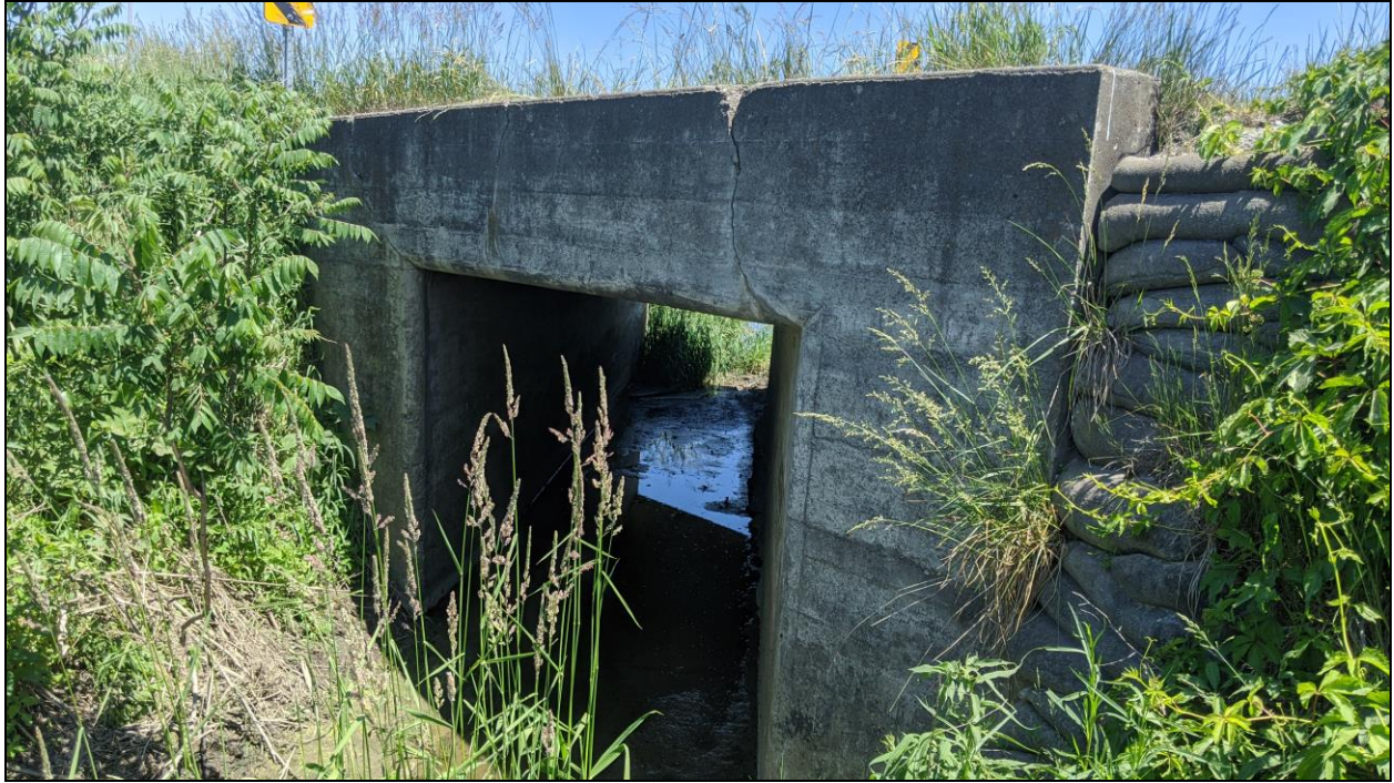
Figure 2. McLarty Line over Fields Creek Drain – North Culvert End, showing structural movement cracking on culvert end wall and fascia, and settlement “concrete bag” retaining walls.
