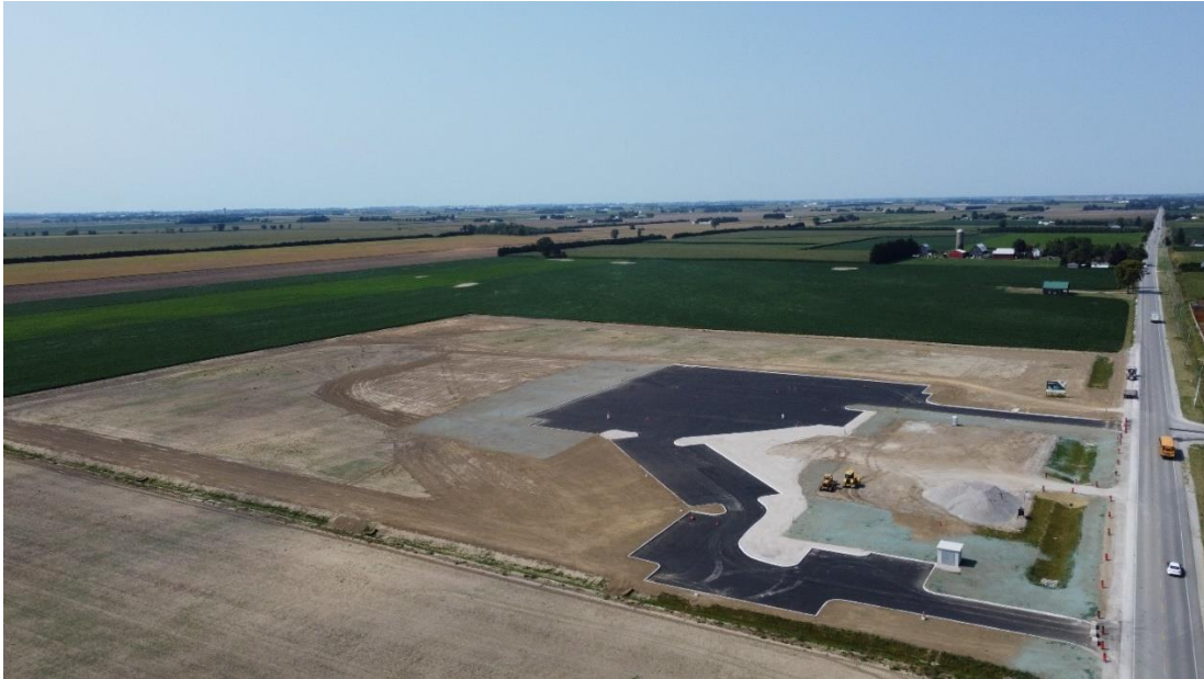
Figure 1 – Drone photo of the park during Phase 1 construction.
