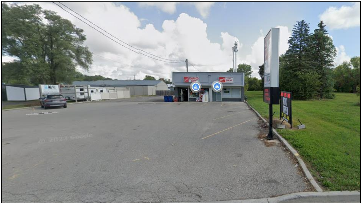
Looking northeast at the subject property.
